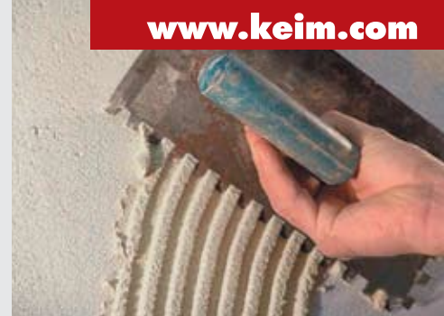
2 notched trowel application of top render layer
