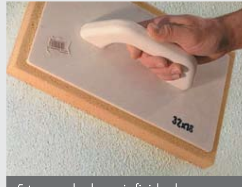
5 top render layer is finished smooth with fine sponge float
