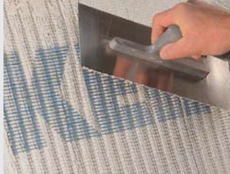
1 bedding the glass mesh by trowel into wet surface of base render
