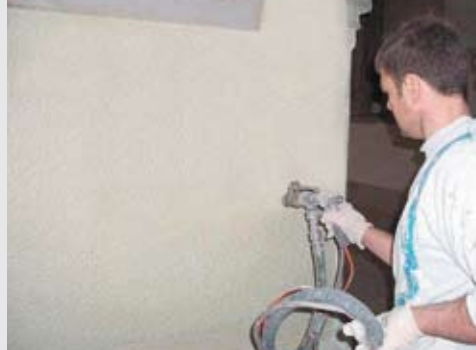
KEIM UniversalPutz renders may be spray applied or trowel applied
