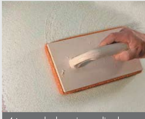
4 top render layer is equalized with coarse sponge float
